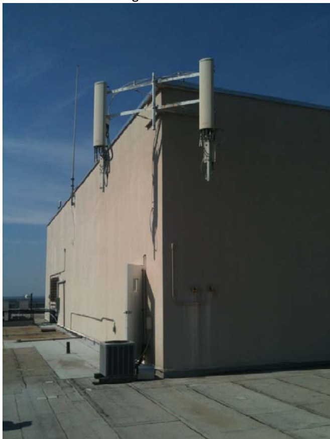
Penthouse – NE View – looking South
