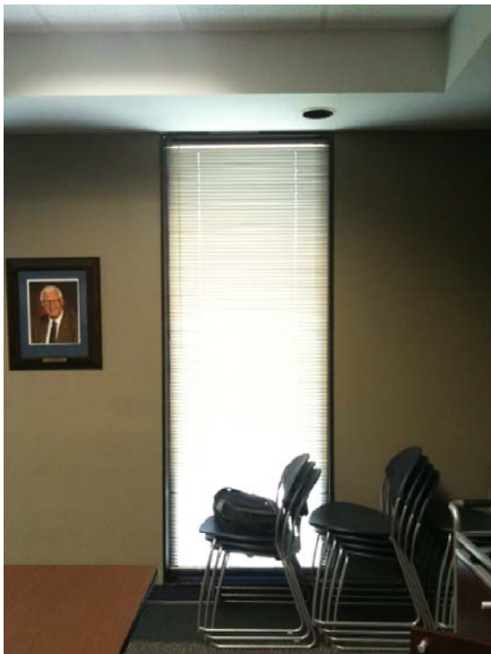
3 rd Floor – Clerk of Courts – Sill Detail: Vinyl Base; Jamb Detail: G.W.B./Painted
