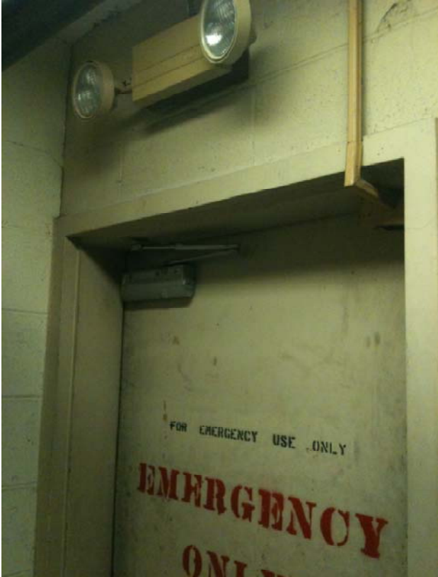
Stair Exit Discharge door detail
