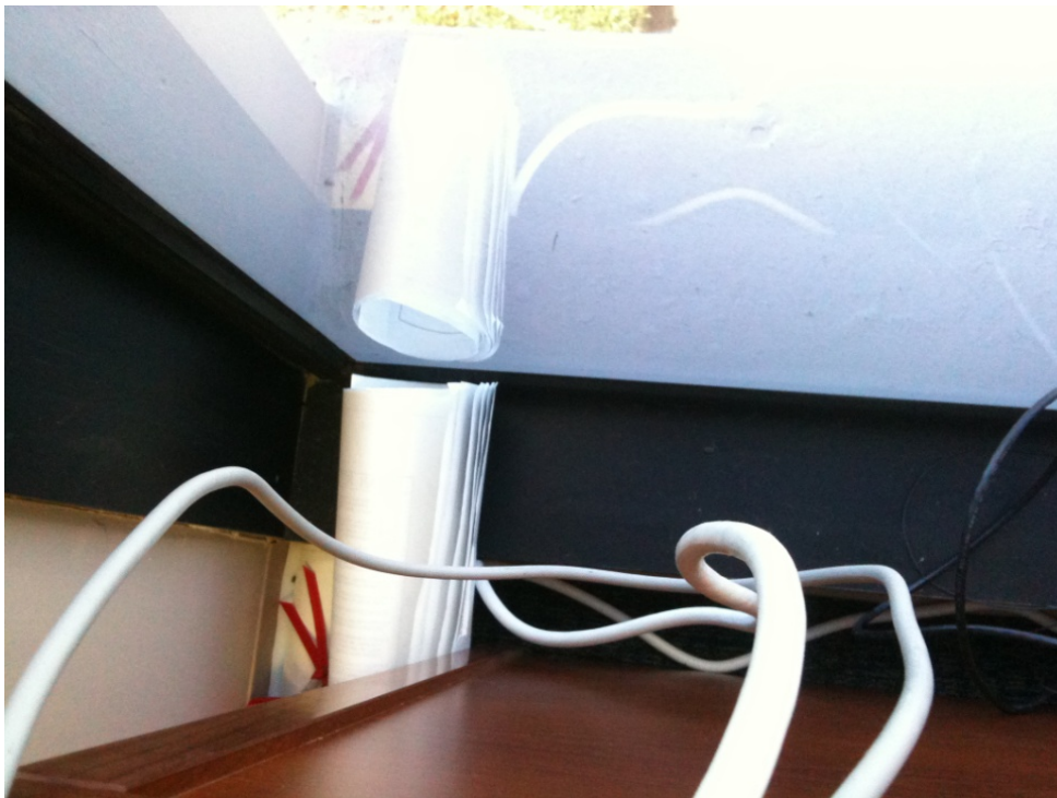
1 st Floor South LC Supervisor of Elections Sill Detail: Vinyl Base
