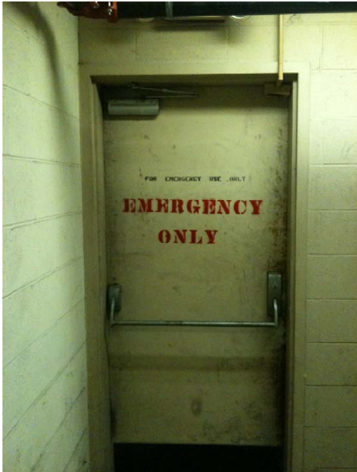
Stair Exit Discharge at Level P-2
