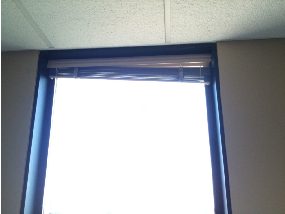
8 th Floor Head Detail: A.C.T. ceiling; Walls - Painted
