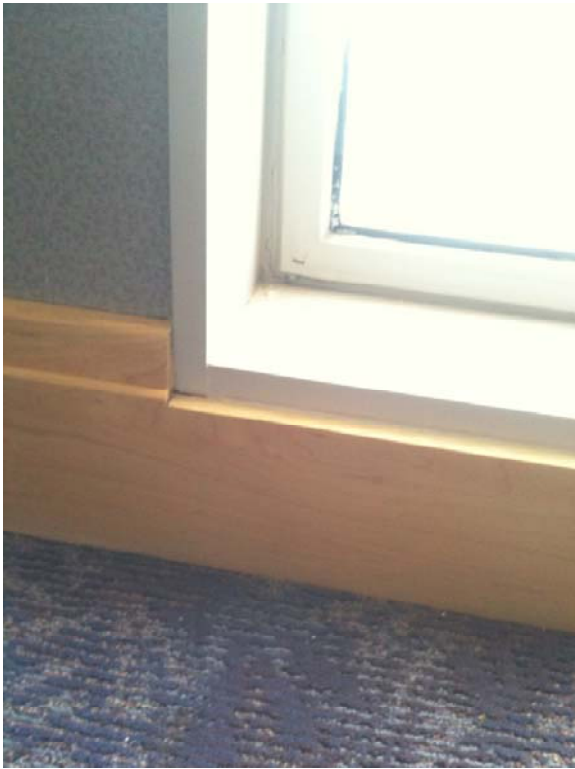
7 th South – Vacant – Sill Detail: Wood Base –stained; Carpet; Walls: Wall Covering;
