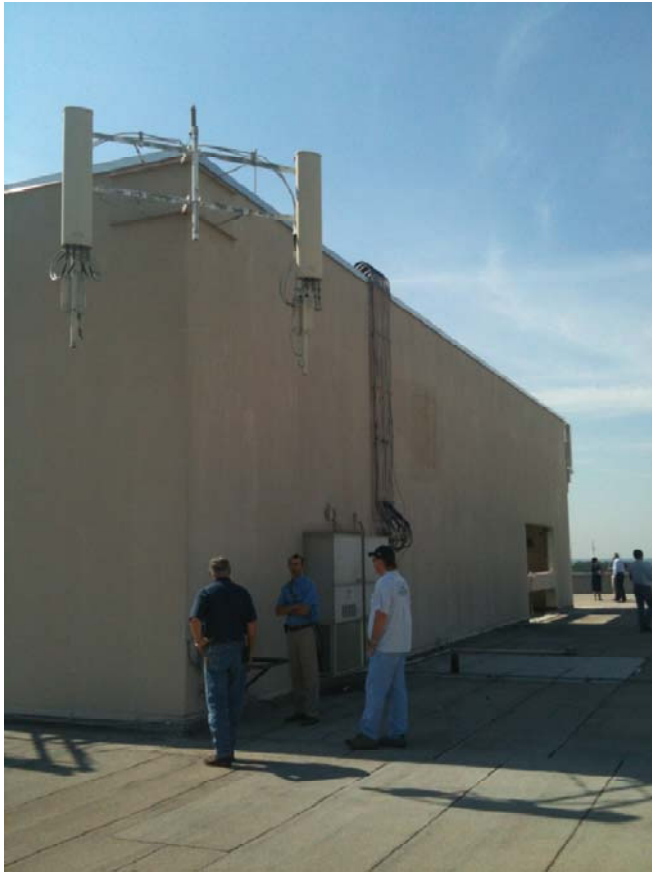
Penthouse – NW View – looking South
